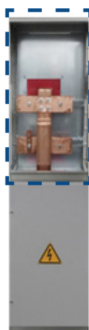
Busbars Compartment Scomparto Sbarre Omnibus
