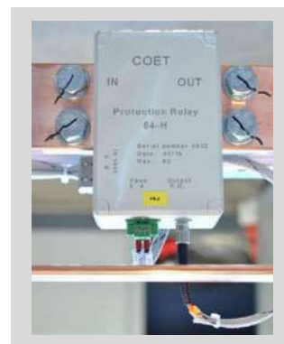
Hall Effect sensor Sensore ad effetto Hall (OPTIONAL)
